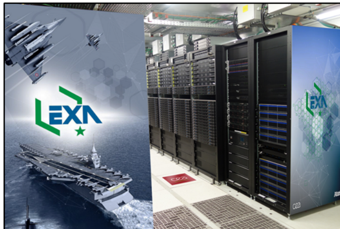
EXA1, centre DAM Ile de France
