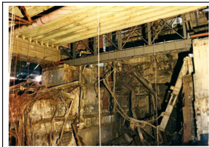
Figure 11 : Poutres supportant le sarcophage
