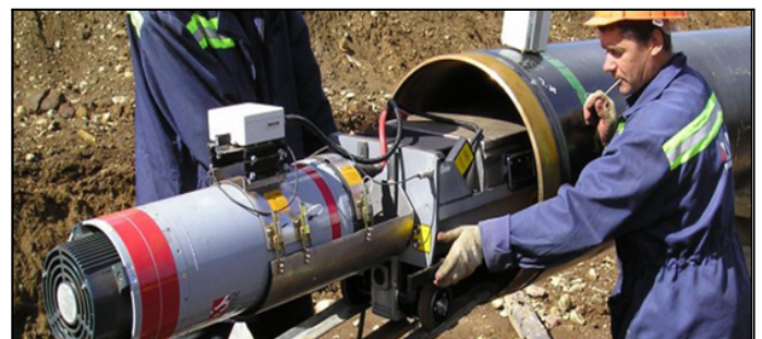
Gamma crawlers © Source JME-Advanced Inspection Systems
